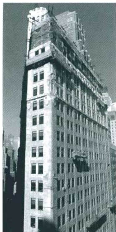
PHOTO: Over 100,000 lbs. of PUMP-X53 were pumped into wall cavities between terra cotta and rubble masonry back-up on this building on Wall Street in New York City as part of a masonry stabilization project.
