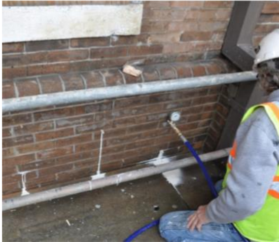
Photo: Pumping PUMP-X53iL with a low pressure grout pump (<30 psi)
