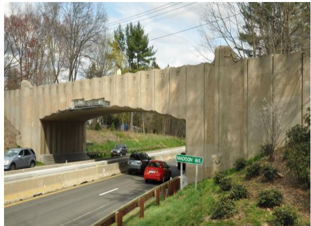
Photos: The Madison Avenue Bridge on Connecticut's National Landmark Merritt Parkway had repair sections form and poured using REPLIC-8. Mix designs were developed from petrographic analysis of core samples and custom color matched.
