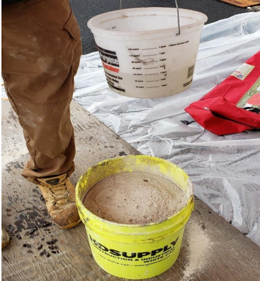
Step 1: Measure the exact amount of clean mixing water for a 60 lb bag of Replac-8 . (Amounts vary based on mix design and weather conditions)
