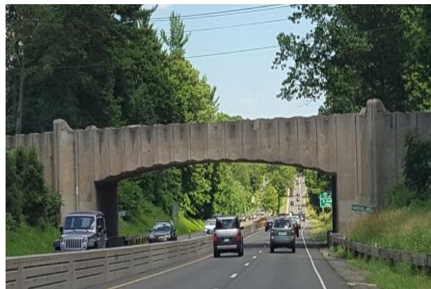
Photos: The Madison Avenue Bridge on Connecticut's National Landmark Merritt Parkway had repair sections form and poured using REPLIC-8. Mix designs were developed from petrographic analysis of core samples and custom color matched.
