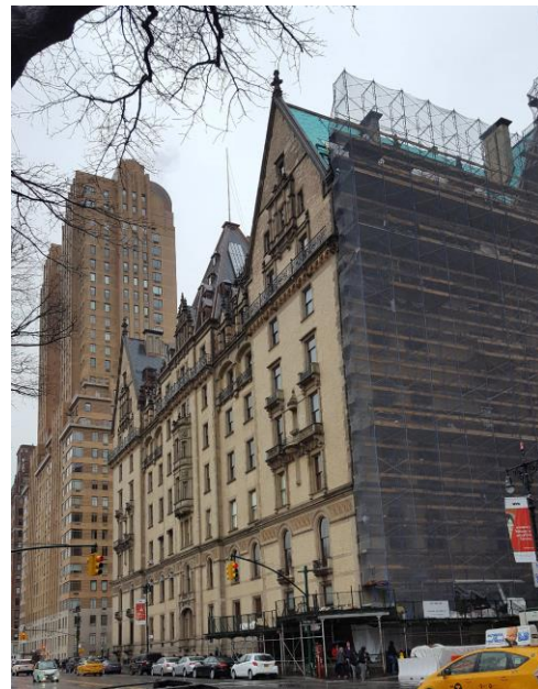
Dakota Apartments, New York City Repointed with Edison NHL 3.5 Mortar
