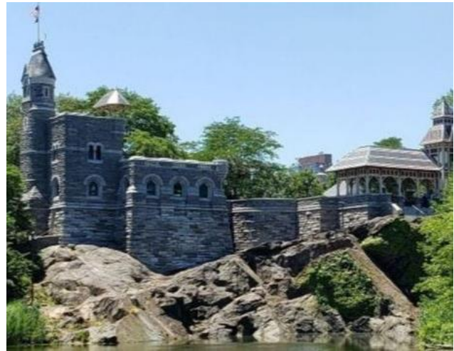
Photo: Belvedere Castle, NYC. E-NHL 50M was used for full repointing of the granite.
