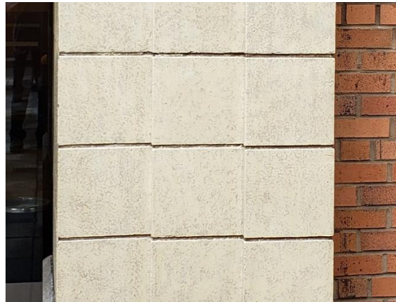
Washing a multi-color Aquathane UA210 terra cotta glaze coating with E-Wash 30 refreshes the appearance without damaging the coating.
