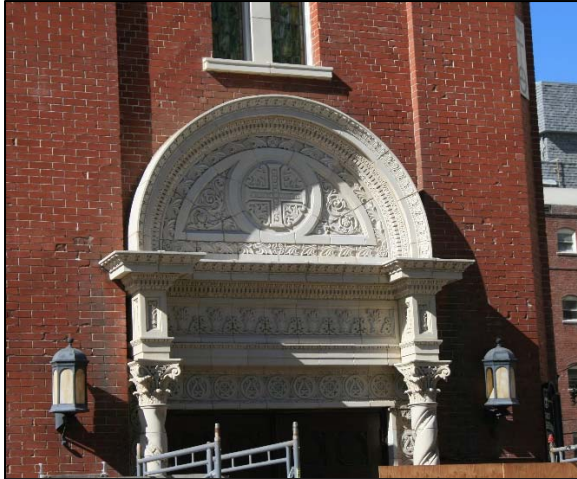
Tower porch cleaned and patch repaired
