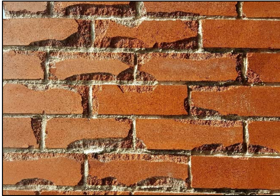
Spalled brickwork
