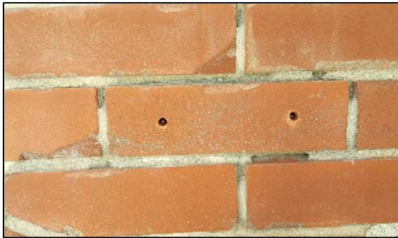
Counter-sunk helical friction anchors installed
