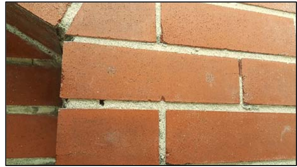
Countersunk anchor holes patched
