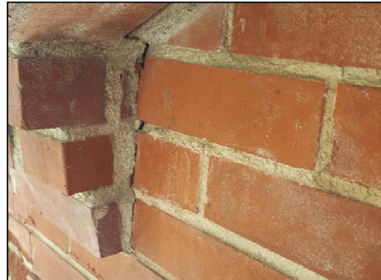
Rotating corbel bricks supporting the faux machicolations and overhanging gable.
