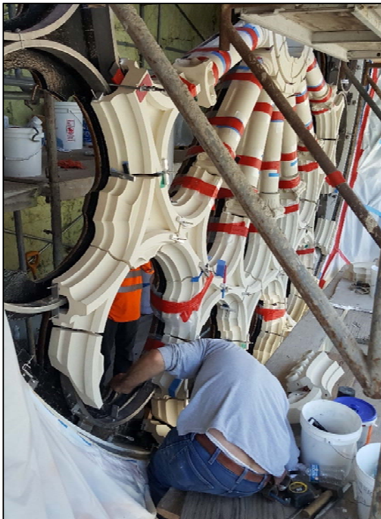
Master mason Shawn Tibbs installing units
