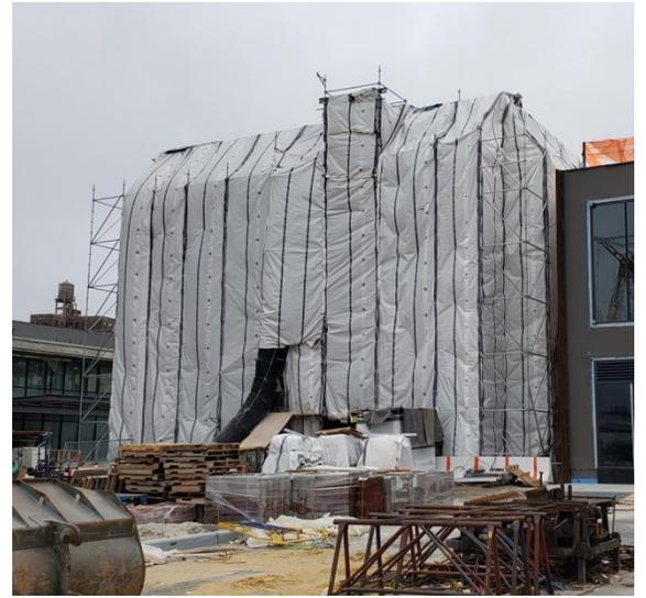
Figure 6. Parapet wall rebuilding in progress using custom-matched BioMix 35
