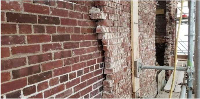
Figure 4. Large sections of the outer wythe were removed and rebuilt.
