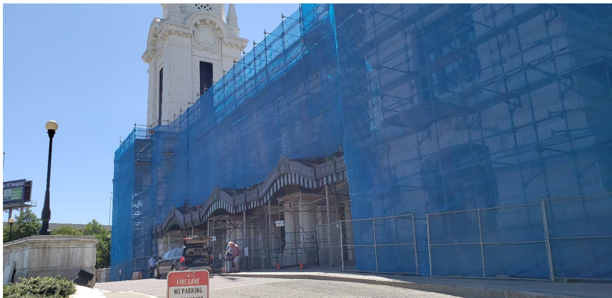
Figure 4. January 2019, a second major restoration in progress
