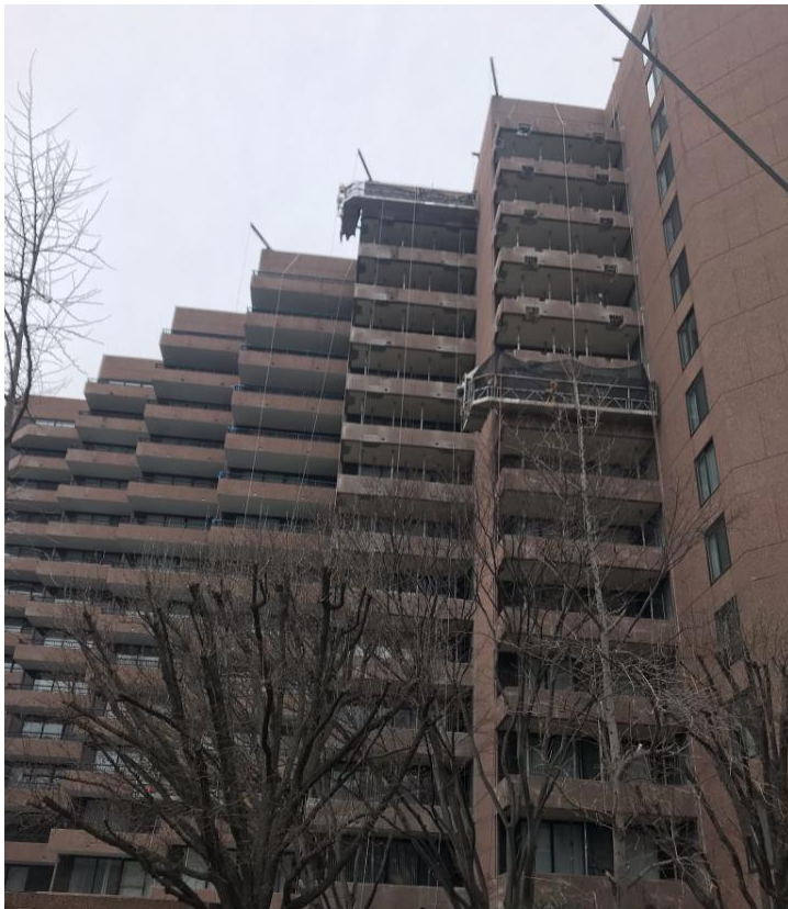
Photos: Mockup panel, above. Custom-matched exposed aggregate repairs utilizing REPLIC-8, left. The two scaffold drops on the right are in progress. The four drops to the left are completed. Courtesy Atlantic Co. Of America.
