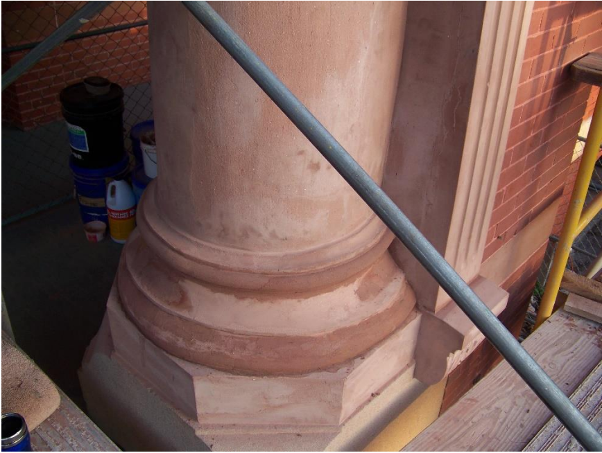
5. Column base repair, in progress
