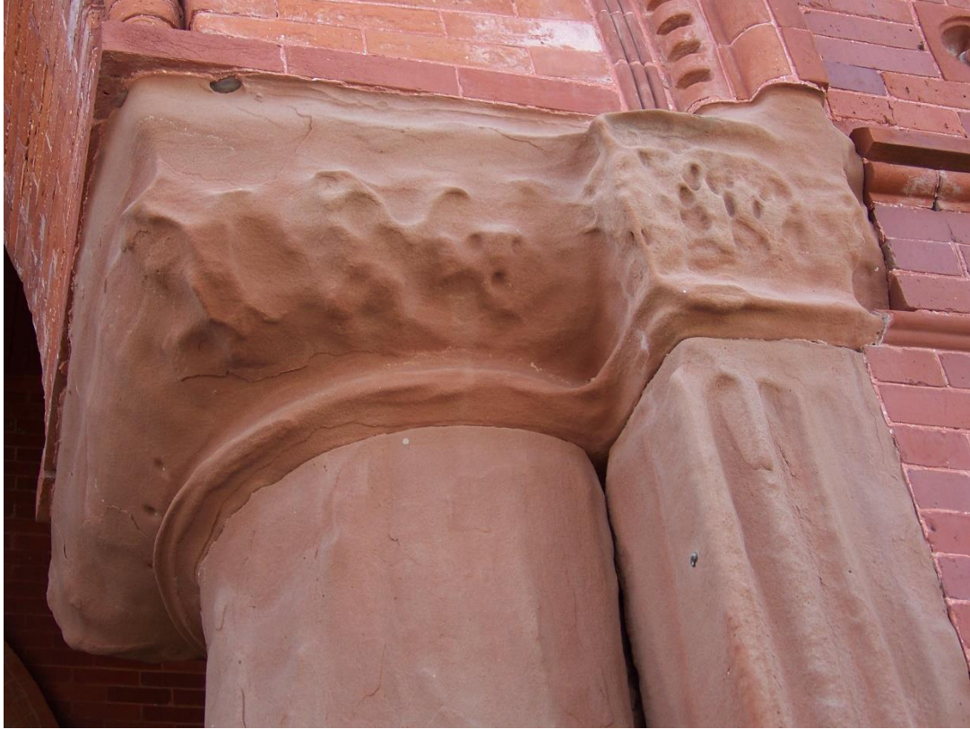
2. Sandstone column, before repair
