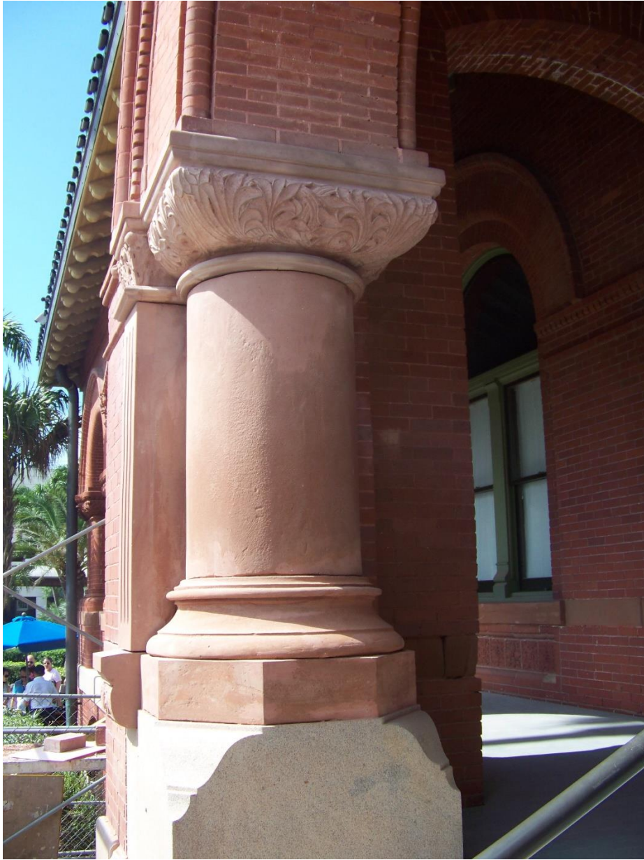
6. Completed column repair
