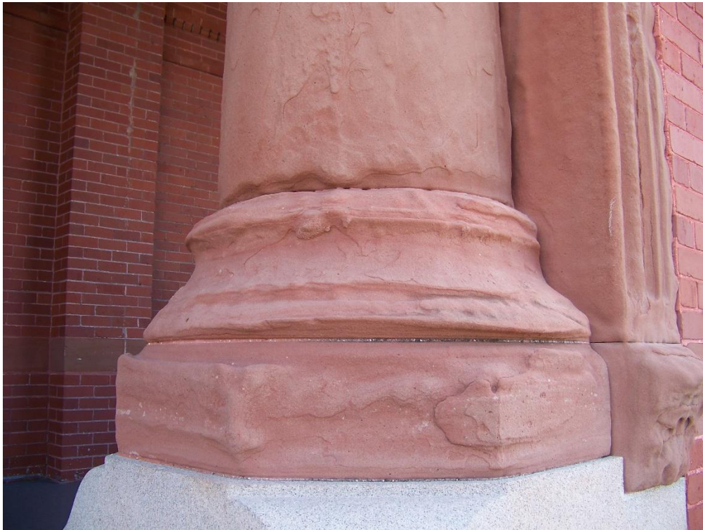
3. Column base, before repair
