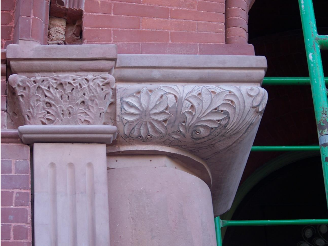
4. Column capital repair, in progress
